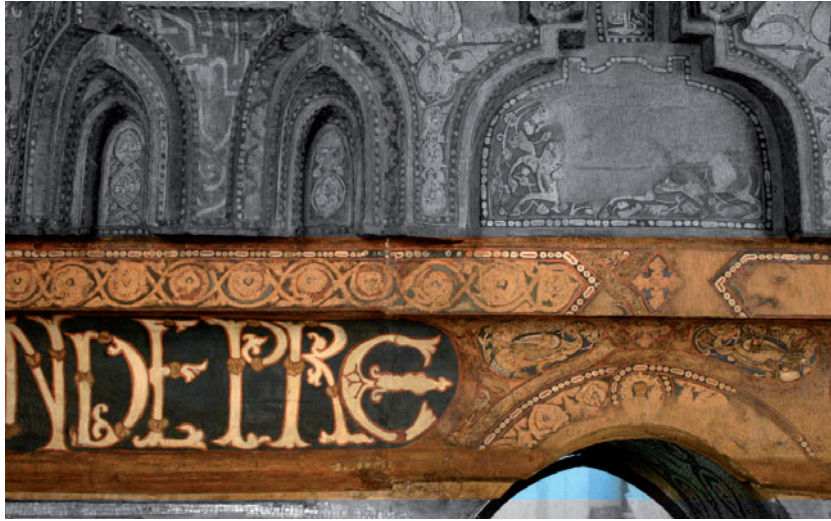
Fig. 8. The molding (in color) at the base of the ceiling. Over the molding is the first tier of the muqarnas frame. The lower edge of the molding fixes the higher end of the mosaic decorations on the walls of the nave; the windows that let light into the nave intersect with the molding. (Photo: Maria Antonietta Badalamenti and Domenico Carbone)
