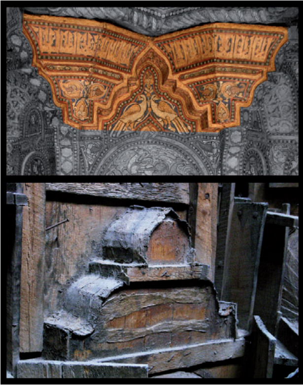
Fig. 53. Fifth tier: the intrados (above) and extrados (below) of the polygonal arch. In the image of the intrados, the big pendentives are clearly visible. (Photo of the intrados: Maria Antonietta Badalamenti and Domenico Carbone; photo of the extrados: courtesy of Arch. Mario Li Castri)
