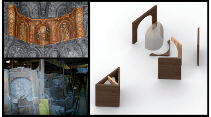
Fig. 46. Fourth tier. Above, left) Flat and cylindrical niches. Below, left) The extrados of the cylindrical niche is highlighted in yellow. Right) Constructive layout of the cylindrical niche. (Image: Fabrizio Agnello and Maria Antonietta Badalamenti; photo of the intrados: Maria Antonietta Badalamenti and Domenico Carbone; photo of the extrados: courtesy of Arch. Mario Li Castri)
