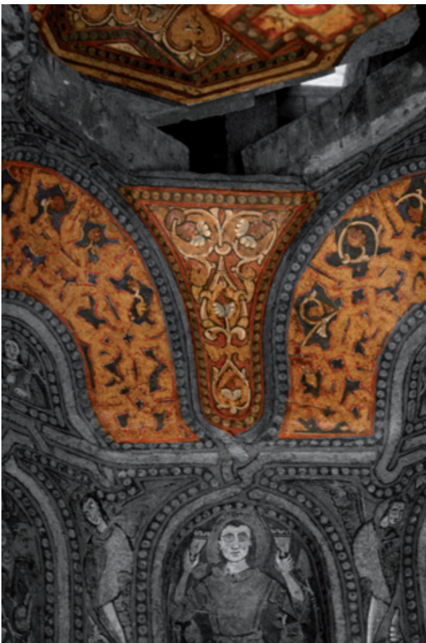
Fig. 49. Fifth tier: the pendentives (highlighted in yellow) that make the transition between the squares and the octagons (“Oc”) (highlighted in dark red). (Image: Fabrizio Agnello and Maria Antonietta Badalamenti)
