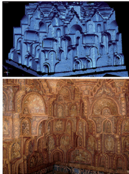
Fig. 10. The ceiling of the nave of the Cappella Palatina, Palermo: northeastern end, detail of 3D laser-scanning data (above) and photo of the muqarnas frame (below). (Photo and 3D laser scan: Fabrizio Agnello, Maria Antonietta Badalamenti, and Domenico Carbone)
