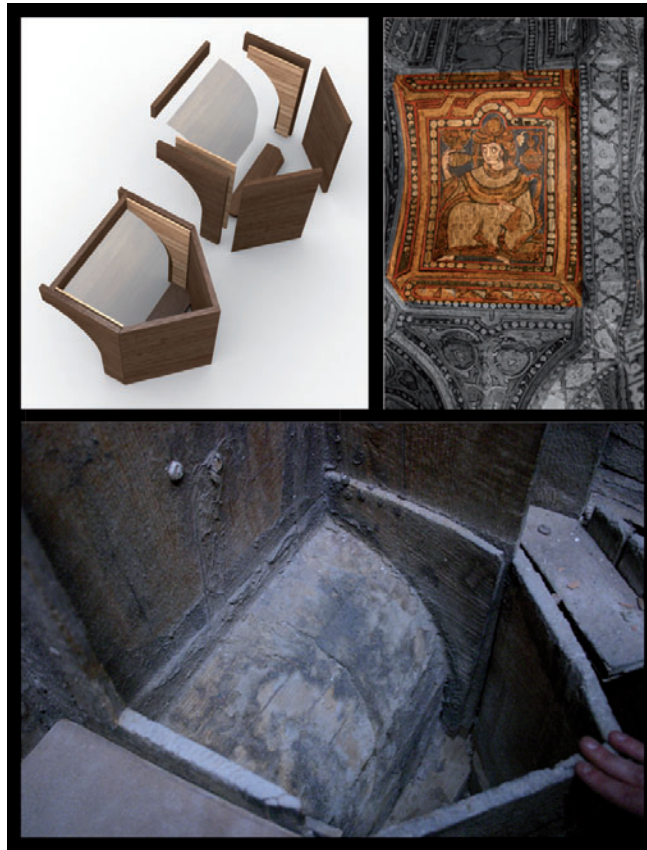
Fig. 38. Third tier: barrel vault. Above, left) Layout of the constructive elements. Above, right) The intrados. Below) The extrados. (Image: Fabrizio Agnello and Maria Antonietta Badalamenti; photos of the intrados: Maria Antonietta Badalamenti and Domenico Carbone; photo of the extrados: courtesy of Arch. Mario Li Castri)
