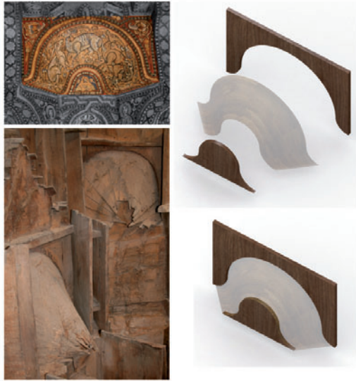
Fig. 45. Fourth tier: constructive elements of the conical vault. (Image: Fabrizio Agnello and Maria Antonietta Badalamenti; photo of the intrados: Maria Antonietta Badalamenti and Domenico Carbone; photo of the extrados: courtesy of Arch. Mario Li Castri)
