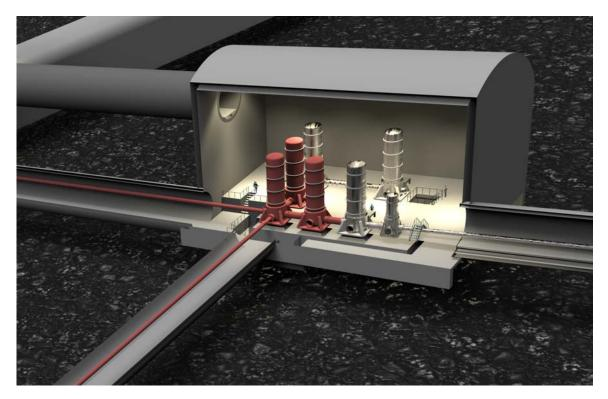
Figure 7.14: CAD rendering of a birds view of cavern B. The entrances to the basement underneath the vacuum towers and a few people for comparison in size are shown.
