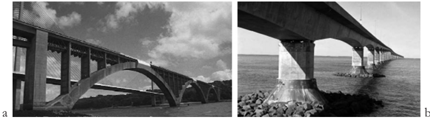
Fig. 4 – a) Ponte ad arco Plougastel (E. Freyssinet). b) Ponte a travata in c.a.p. Confederation Bridge (J. Muller)
