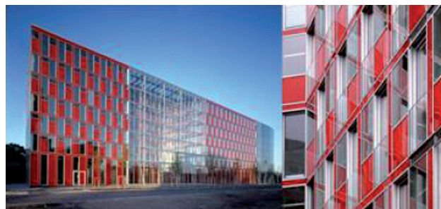
Fig. 1 The DSC-based PV façade of the Capricorn Haus in Germany. (Reproduced from Gattermann und Schossig Architekten, with permission).
