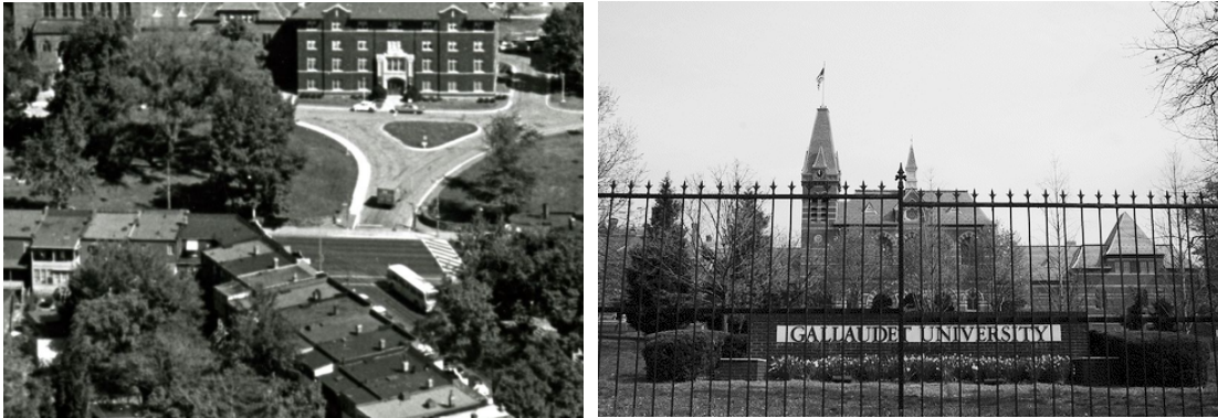
Figure 22: (Left) Aerial View (1965), Before addition of the fence (Source: Gallaudet University Historical Photograph Collection." Gallaudet University. 1965. https://gaislandora.wrlc.org/islandora/object/historicalphotographs%3A1091 (accessed 12 05, 2021)). (Right) Florida Ave. View, After addition of the fence in 1968 (Source: Tozier, Jason. Gallaudet College: The Fence)
