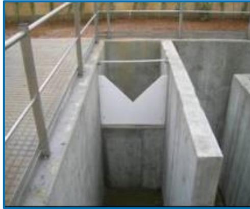
*Figura 1 Vertedero rectangular, triangular y canal Parshall*
