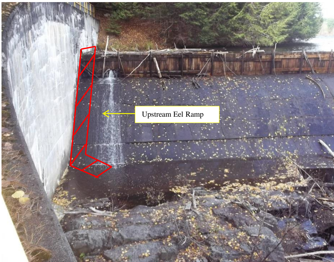
Figure 10. Conceptual design of upstream American eel passage facility at Weldon Dam. (Source: GLHA, 2015).
