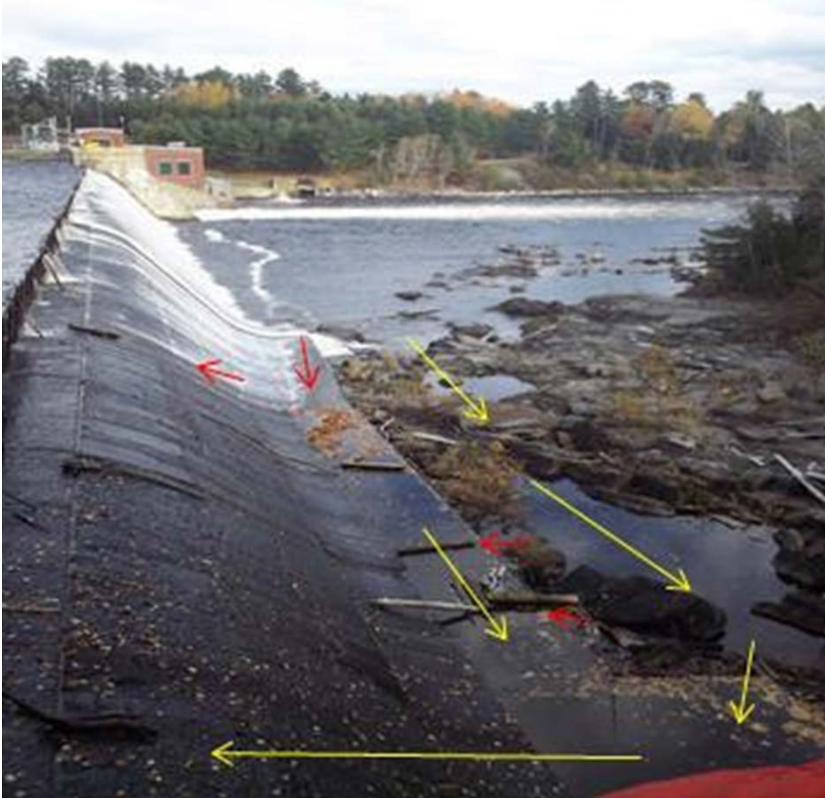
Figure 9. Upstream American eel migration routes for Weldon Dam. Arrows indicate upstream eel migration routes: yellow arrows indicate the primary upstream eel migration routes and red arrows are secondary routes.
