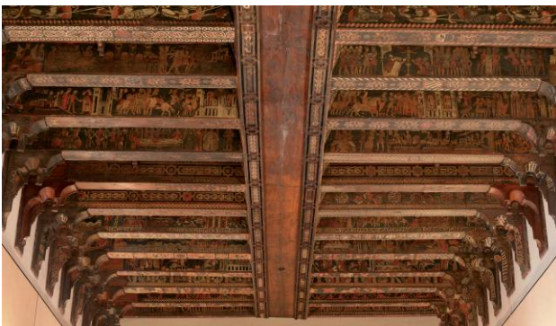
Figure 3. The wooden ceiling of the “Magna” Hall.
