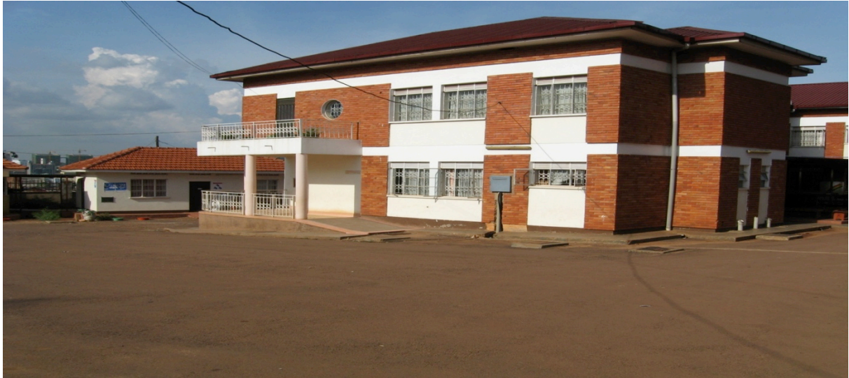
Figure 12: New building for the Home Care Department of Nsambya Hospital (NHC) supported by the TFP.
