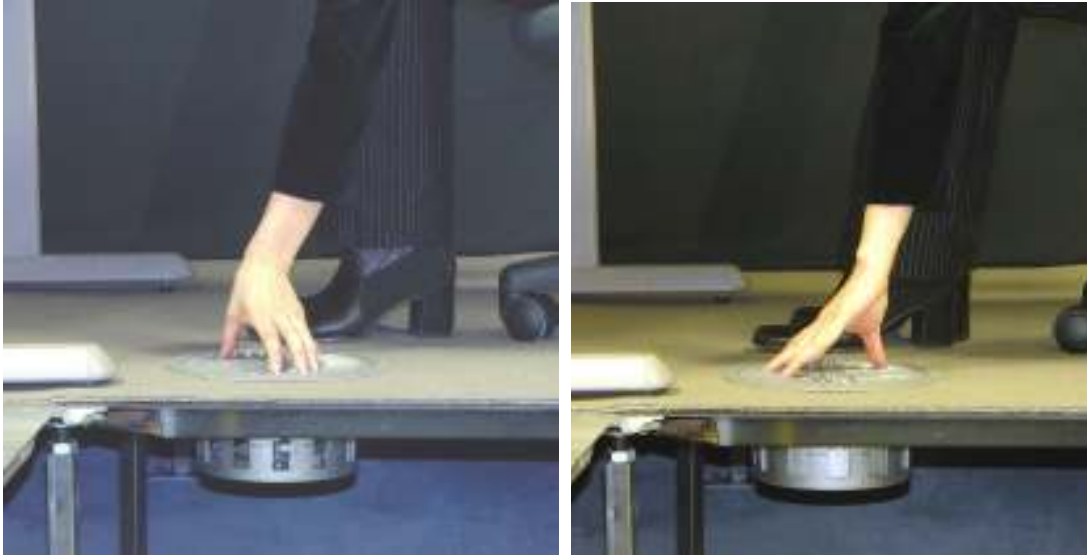
Figure 1-8 Air flow regulation through the diffuser
