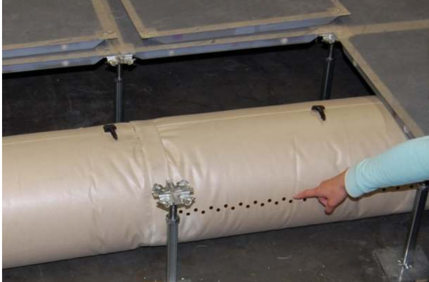
Figure 4-1 Orifices along the duct
