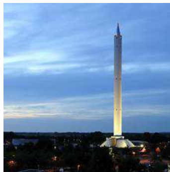
FIGURE 2.5: ZARM drop tower in Bremen (courtesy of ZARM).
