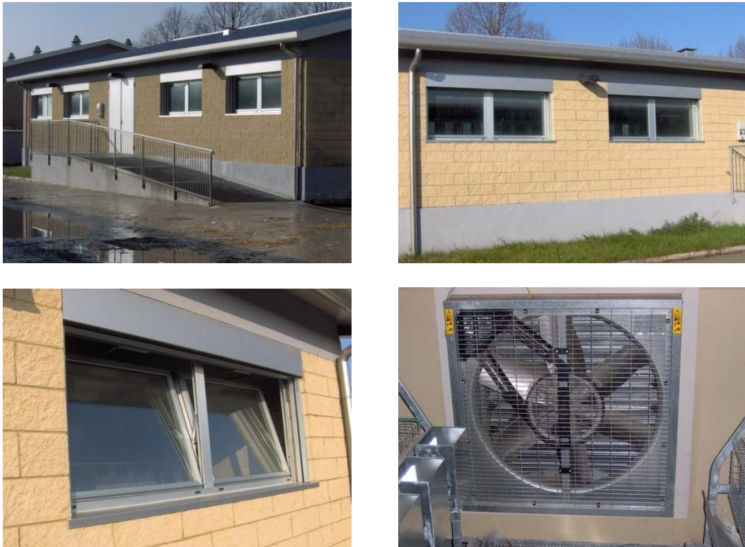
Figure 3. Experimental facilities and equipments for air circulation and extraction fans.
