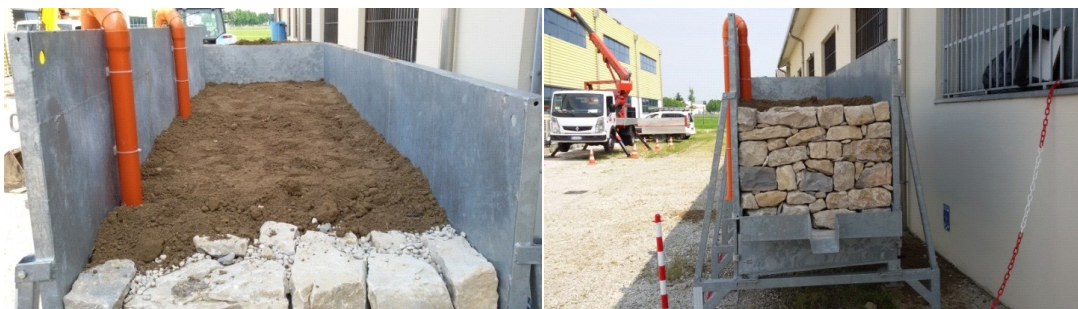
Figure 3.6. the terraced slope completed
