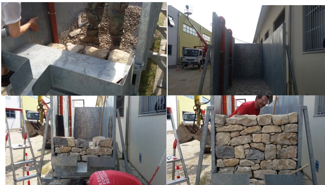
Figure 3.4. Realization of the dry wall
