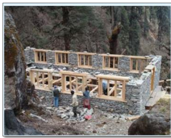
Fig.1. 3b: Building construction
