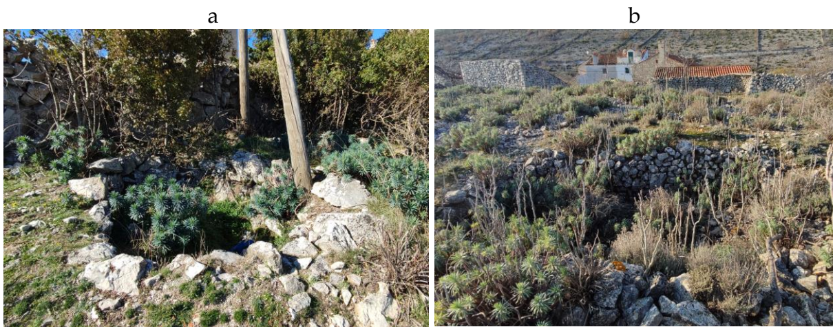
Figure 83. Reservoirs in which lime is slaked can be found on the margins of the villages: a) fòš of Lubenice (2021) and b) fòš of Predošćica (2021)
