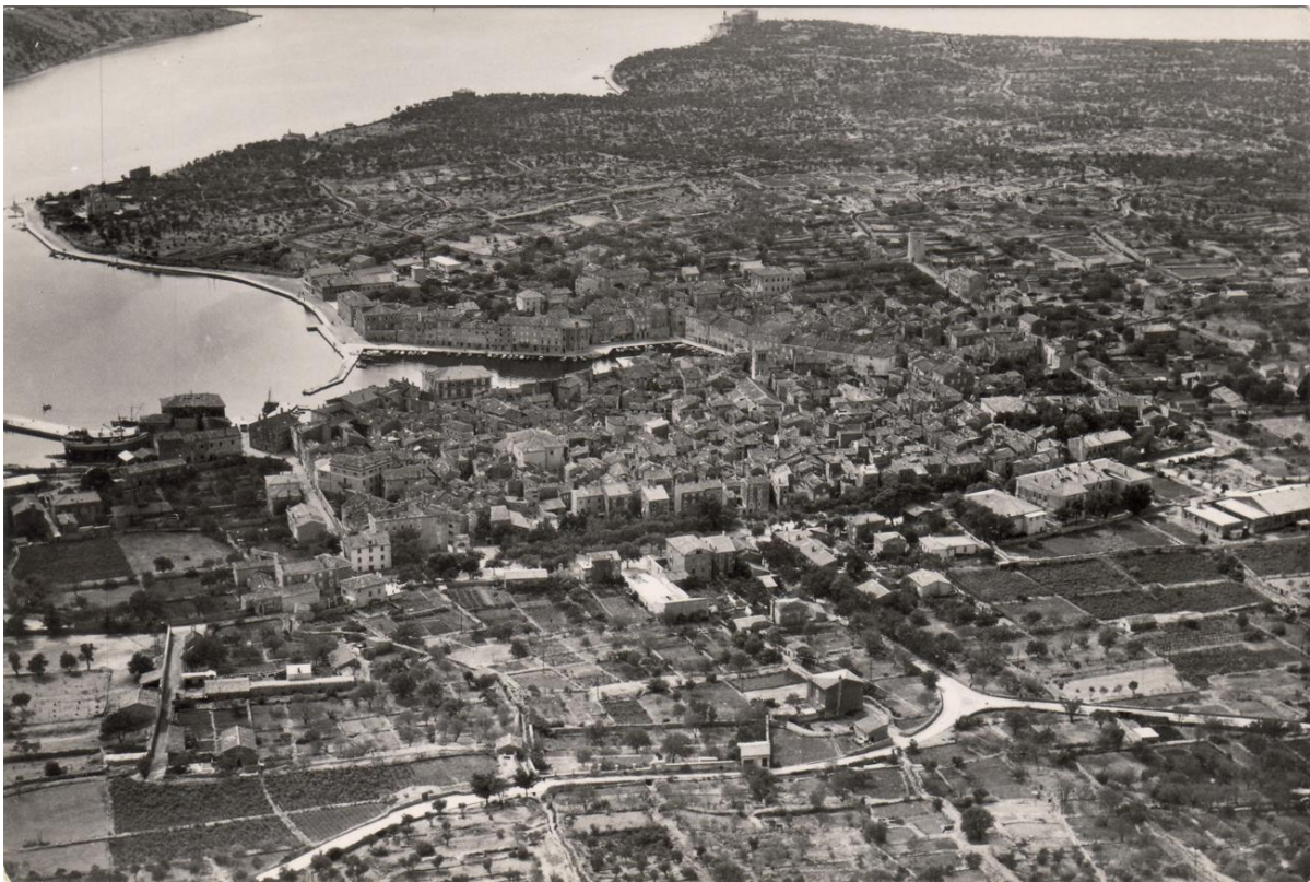
Figure 161. A rare high-quality photograph taken at the beginning of the 20 th century. In addition to the paths that lead from the town to the olive grove parcels, regular orthogonal patterns of arable crop land close to the town are discernible. Today, this ground is mostly used for new house construction. (D. Rendulić - Agencija za fotodokumentaciju Zagreb, 1960s)
