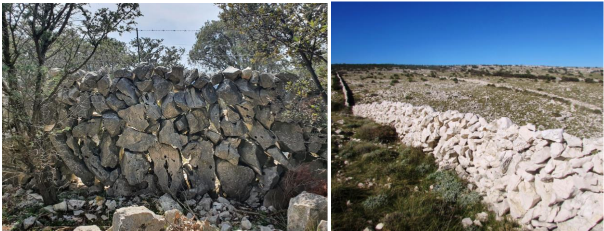
Figure 16. Single walls a) reinforced with wire (2021) and b) on the eastern shores of the island of Cres (2019)
