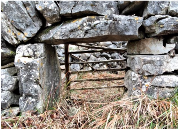
Figure 110. Lunky holes ( škùja ) of a sheepfold closed by a wooden door ( lesa ) in the area of Bagen (2021)
