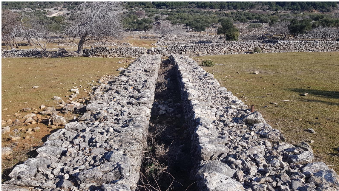
Figure 65. The drainage canal in the fields (Poje, 2019)
