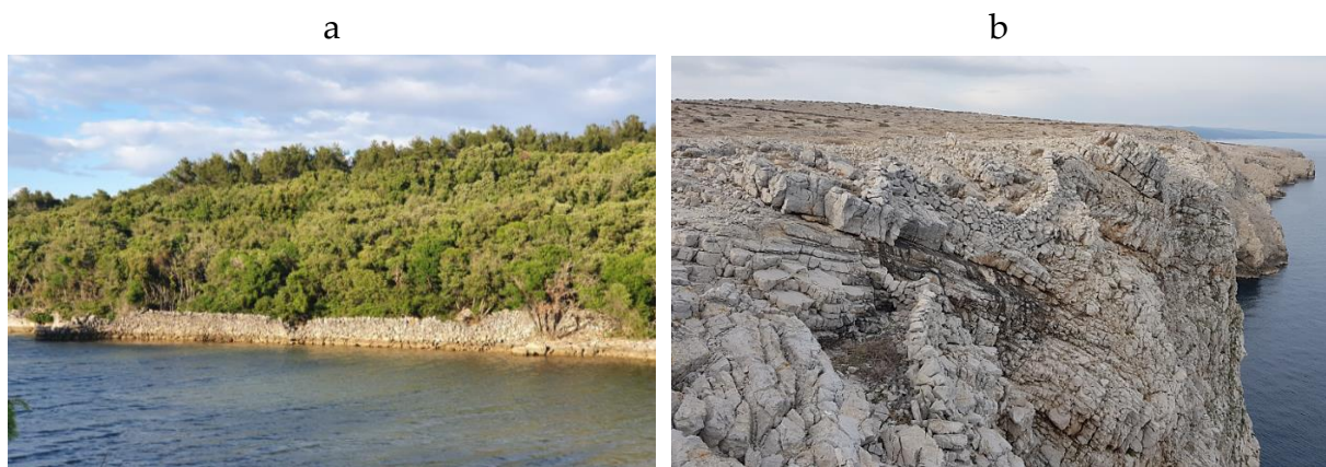
Figure 4. Dry stone walls built all the way to the sea a) on the lower shores of the bay Ul of Punta Križa (2021) and b) on the higher and steep cliff of the eastern shore of the island of Cres (2020)
