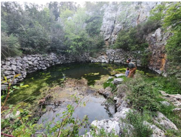
Figure 68. A community pond close to Vidovići, said to never evaporate fully, attached to an escarpment, lined with thick dry stone walls, and containing a paved stair entrance (2021)
