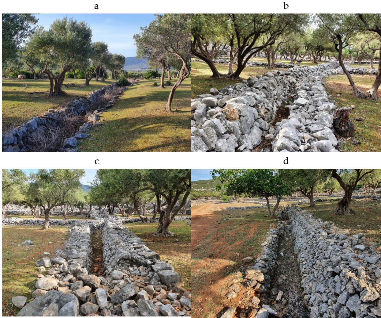
Figure 58. Examples of the well-maintained or well-preserved dry stone canals on the northern slope of the Cres olive grove: a) The canals are frequently used as places to dispose of pruned olive tree branches. b-c) Dry stone canals of thicker construction and c-d) the chamfer mode of construction, found at the margins of a parcel (2020).
