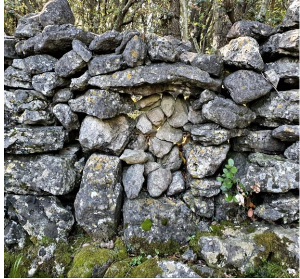
Figure 109. Lunky holes ( škùja ) closed with stones a) on the pathway between Germov and Miholaščica (2021) and b) between Halmac and Veli Tržić (2020)
