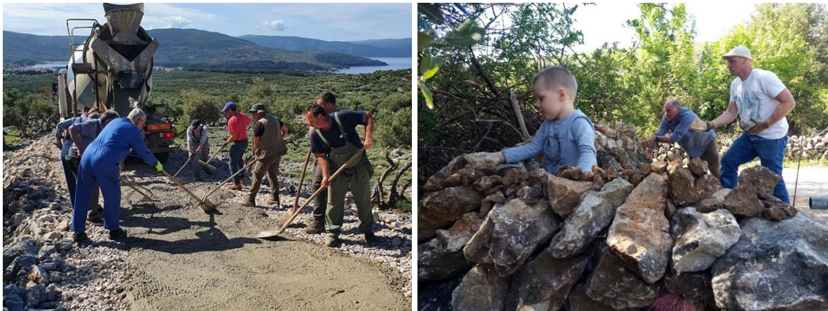
Figure 187. The annual work of the members of the Cres olive growers' association 'Ulika' of concreting the roads to olive groves in order to facilitate agricultural production, but at the expense of the vernacular dry stone architecture (© Franko Fučić)
