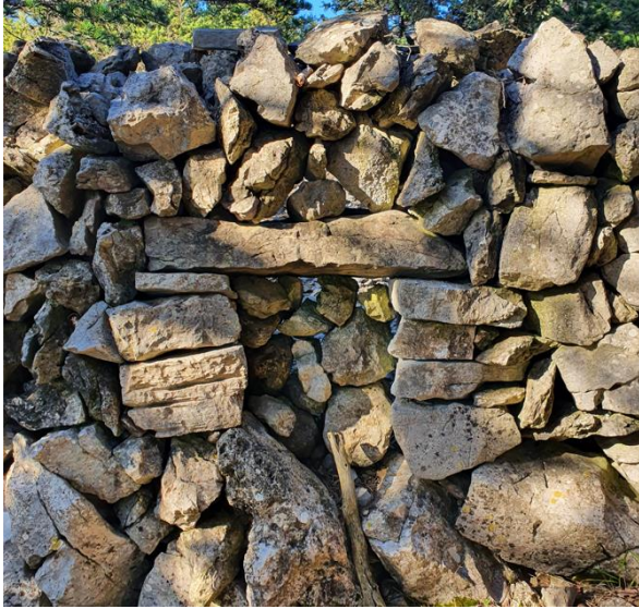
Figure 109. Lunky holes ( škùja ) closed with stones a) on the pathway between Germov and Miholaščica (2021) and b) between Halmac and Veli Tržić (2020)
