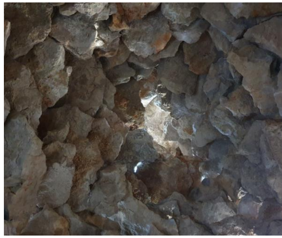
Figure 97. A dry stone corbelled hut in the pine forest close to Pržiči (a-d), located close to the clearance wall, with a roof corbelled with stones and inner bench (2020)
