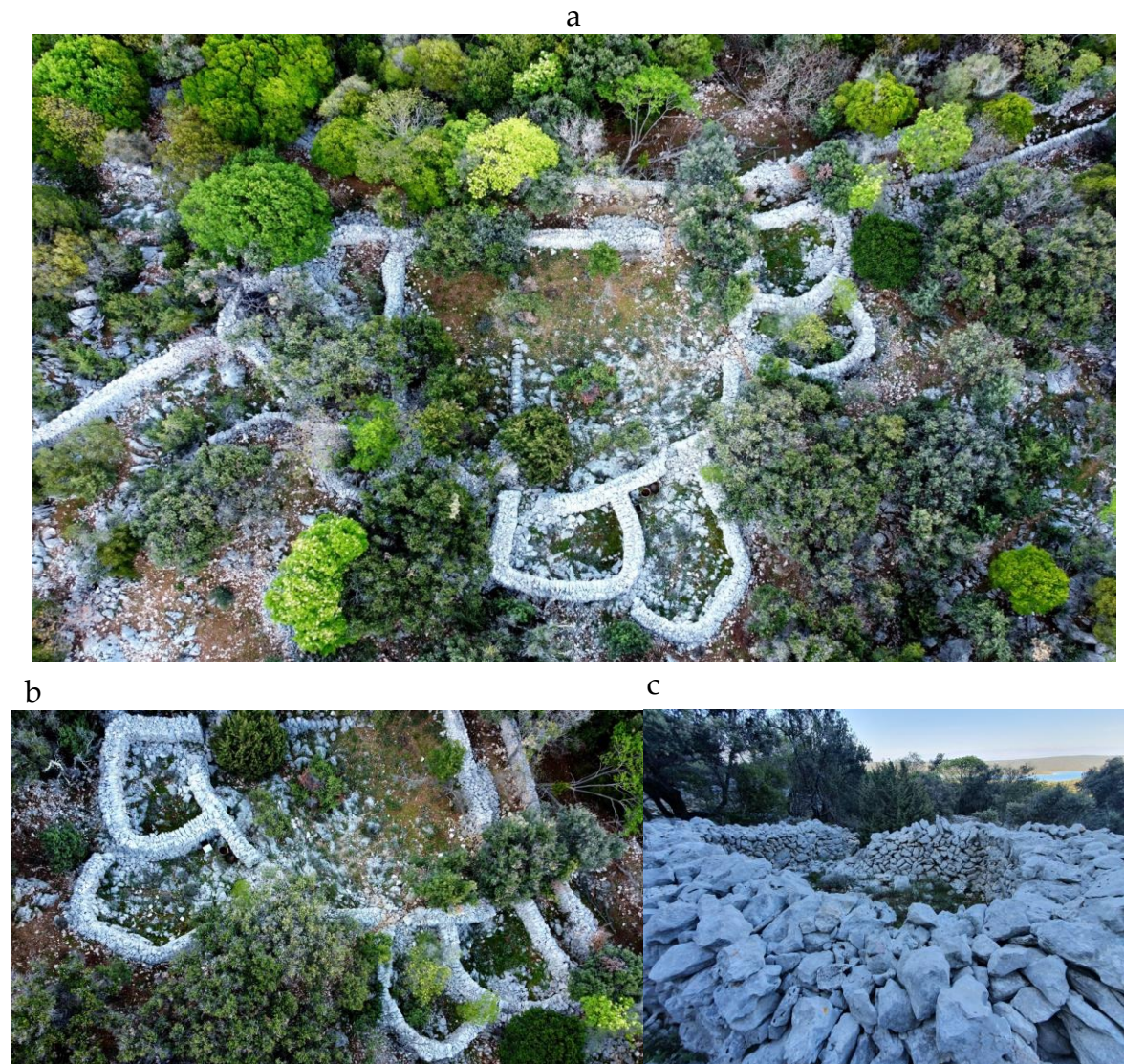
Figure 53. The multicellular, half-flower shaped eight-cell sheepfold close to the abandoned village of Veli Tržić , on the hill Osorščica (island of Lošinj ): a) Full aerial view, b) an image showing that structures are still mostly preserved, and c) an image of one of the sheepfold compartments made with a massive double dry stone wall (2021)
