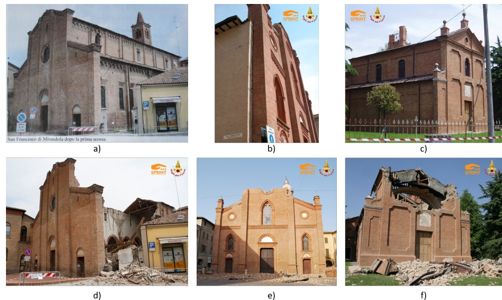
Figure 14. Photos showing the damage of: (a,d) church of San Francesco in Mirandola after the Emilia-Romagna earthquakes of 20 May 2012 (a) and 29 May 2012 (d); (b,e) church of Santa Maria Maggiore in Mirandola after the earthquakes of 20 May 2012 (b) and 29 May 2012 (e); (c,f) church of San Luca in Camurana after the earthquakes of 20 May 2012 (c) and 29 May 2012 (f). The pictures derive from the database of CNVVF-NCP [94], with exception from picture (a) from https://www.italianostramodena.org (accessed on 13 April 2021).
