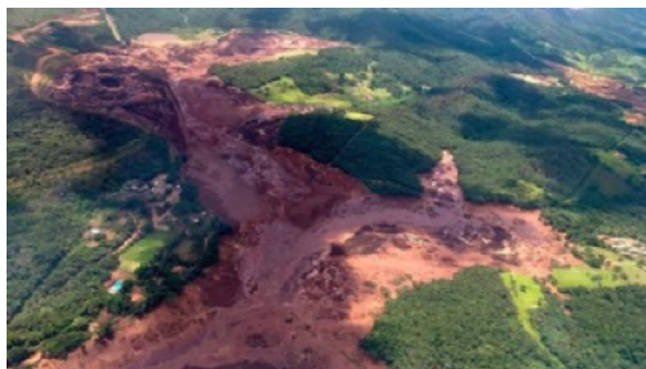
Figure 1.1: Slurry released in Brumadinho dam collapse (25/1/2019, Brazil)
