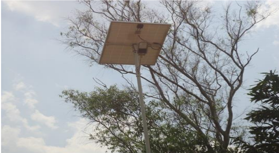
Figure 4.2 Stand- alone PV Lighting System
