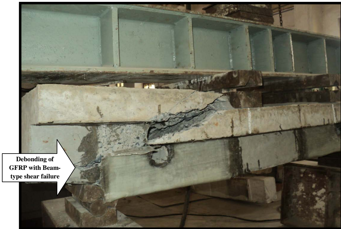
(c) Failure Pattern of SB11 (Beam-type shear failure)
