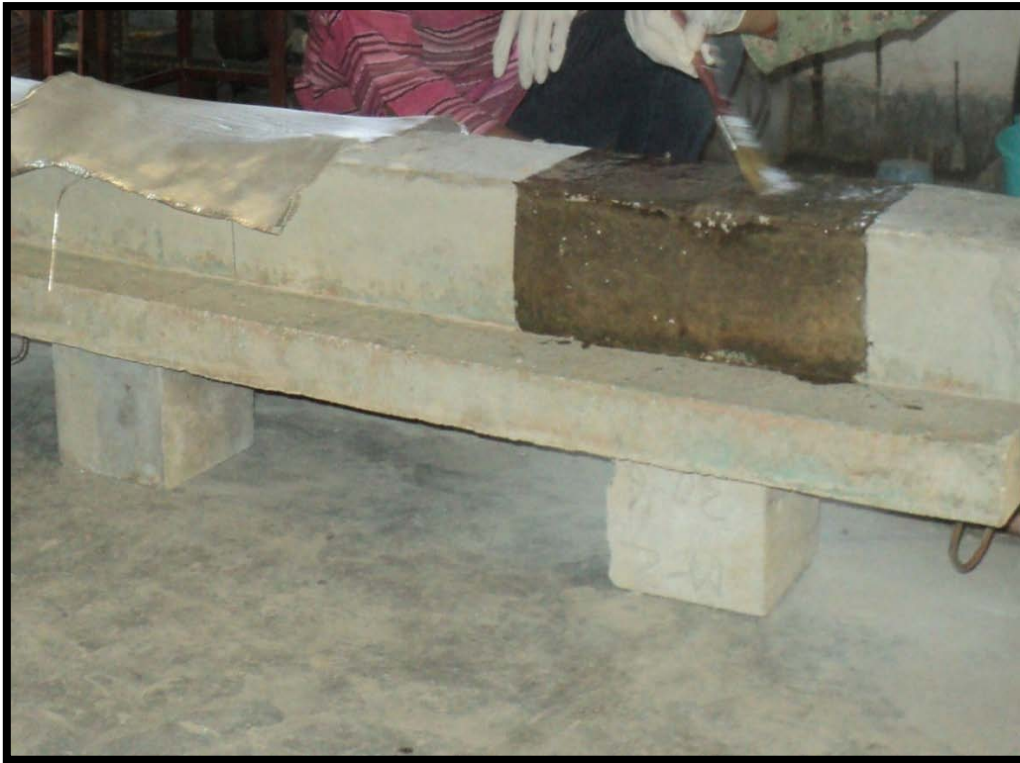
Figure 3-7. Application of epoxy and hardener on the beam
