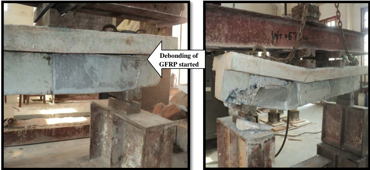
(b) Initiation of debonding of GFRP sheet
