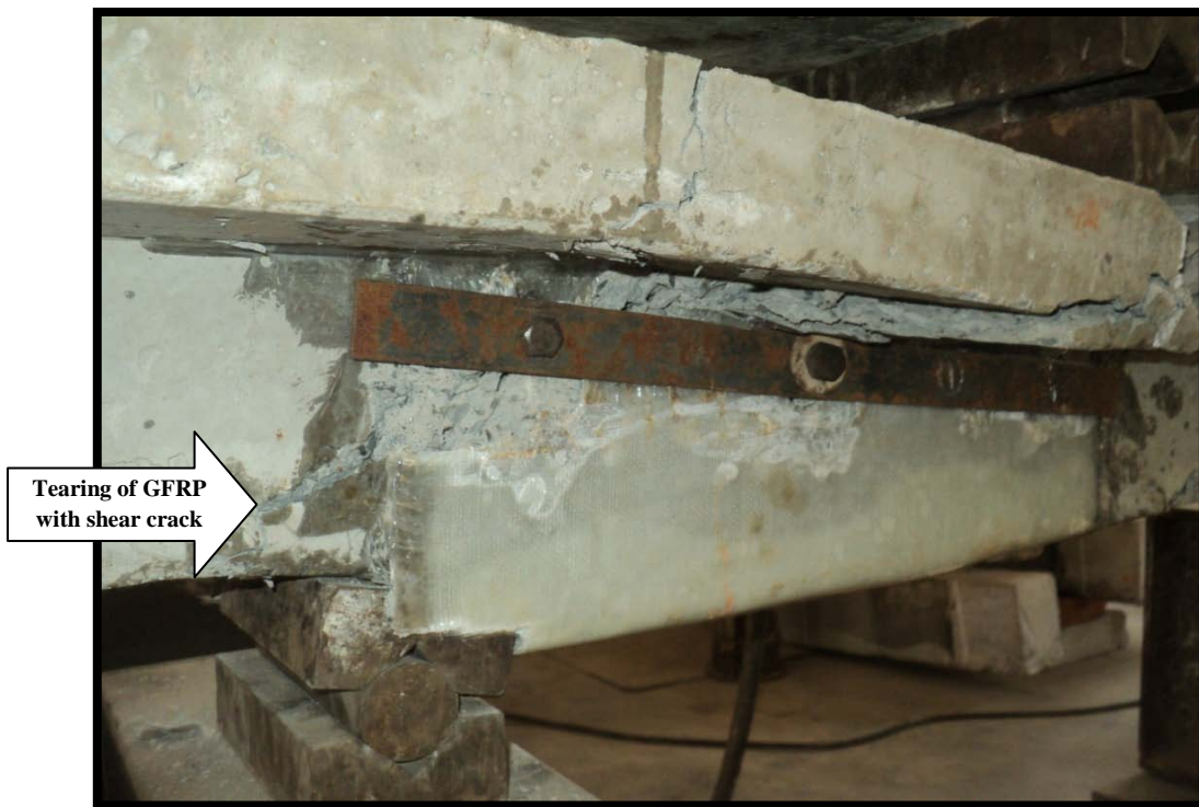
(c) Magnified view of Tearing of GFRP followed by shear failure
