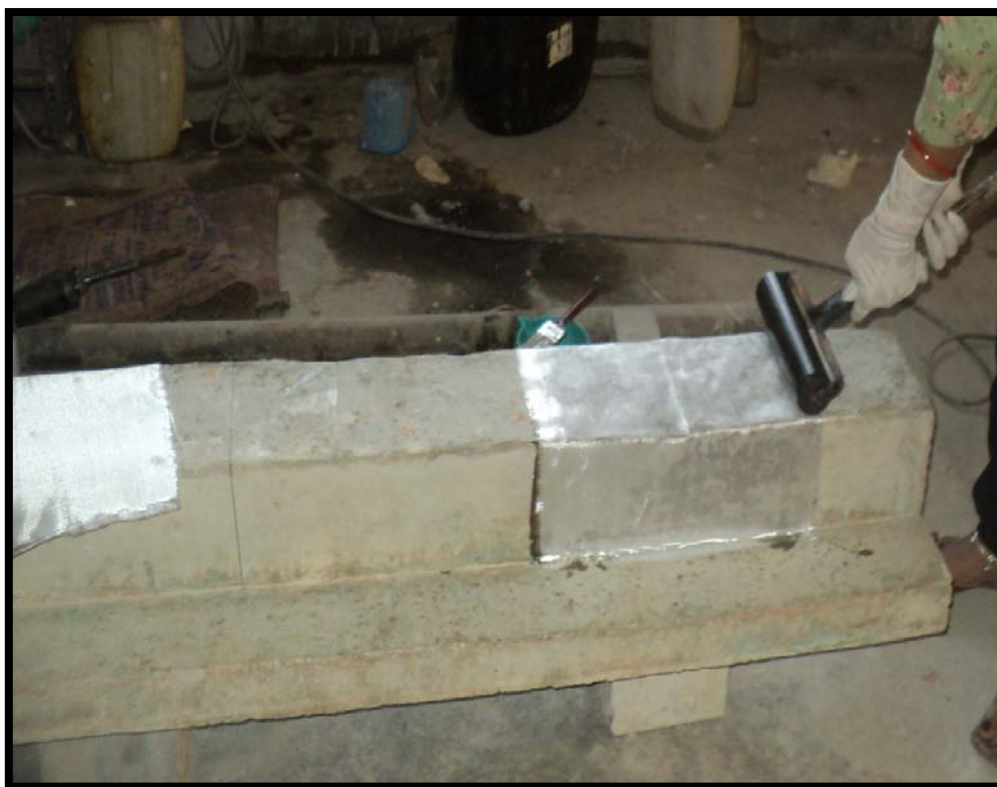
Figure 3-9. Roller used for the removal of air bubble
