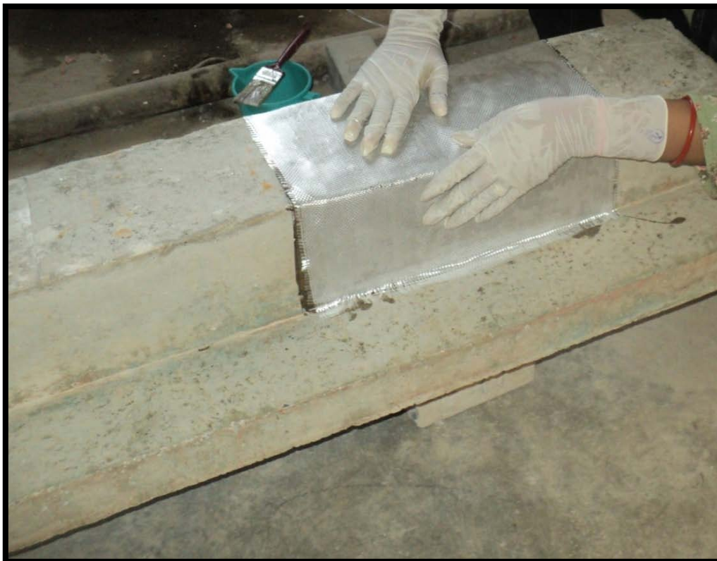
Figure 3-7. Application of epoxy and hardener on the beam
