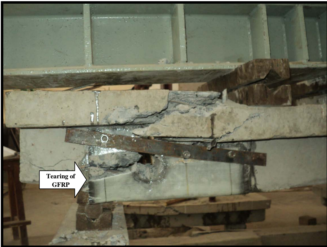
(b) Tearing of GFRP sheet followed by Beam-type shear failure
