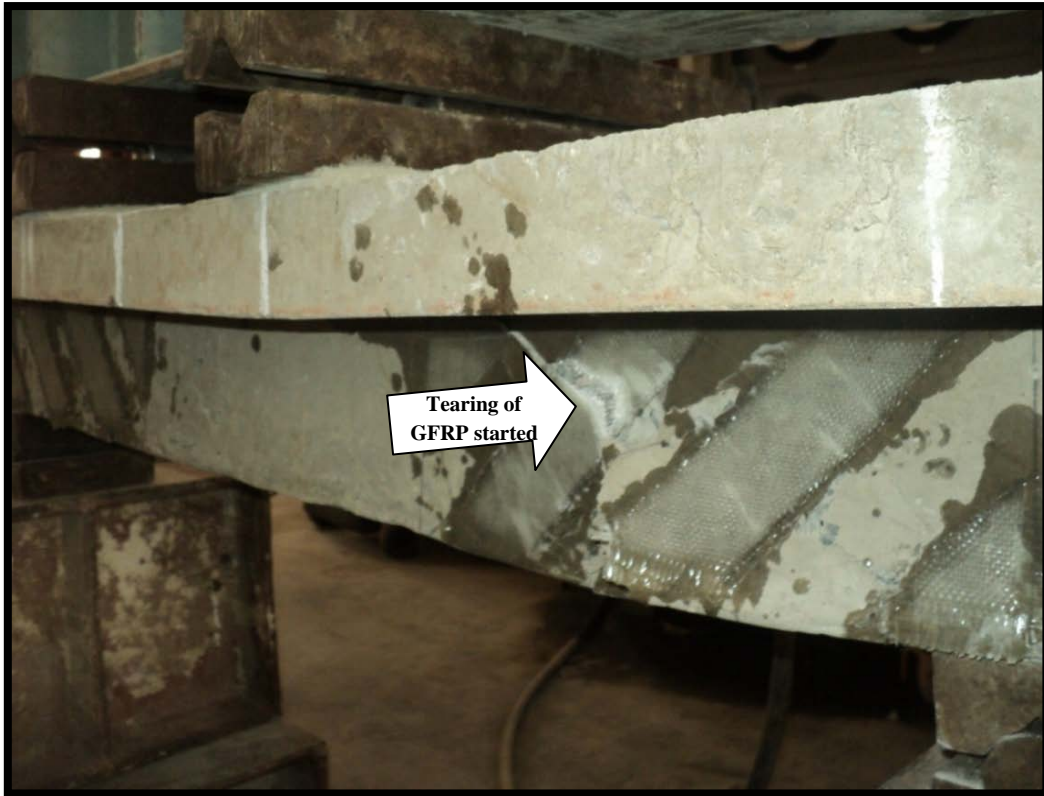
(b) Initiation of tearing of GFRP sheet Started at load of 80 kN
