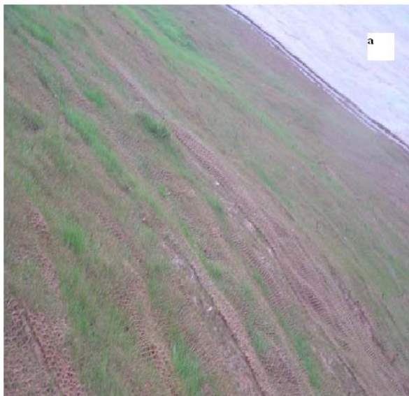
Figure 3 (a) Coir Matting on dump slope
