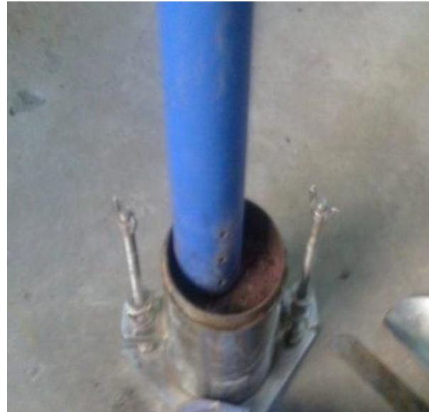
Fig:- 4.2: Application of blows
