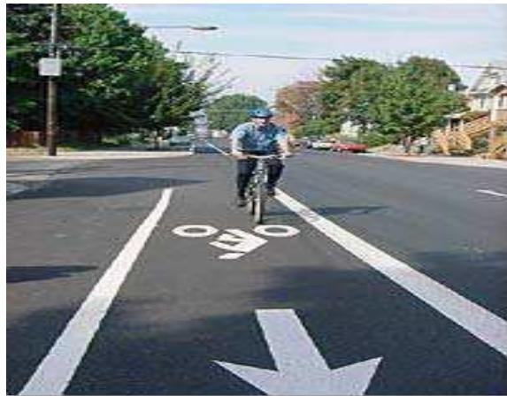
Figure2.2 Represent the designated bicycle lane with pavement marking (Source Developing a bicycling level of service map for New York state )
