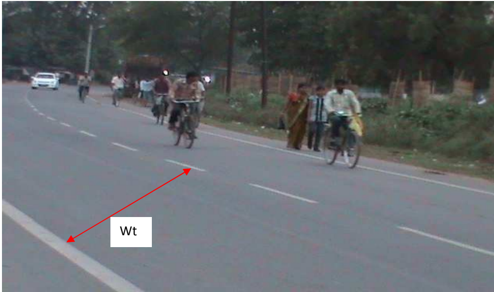
Figure 5.2 Width of pavement for the outside lane and shoulder ( W_t ) (two lane undivided)
