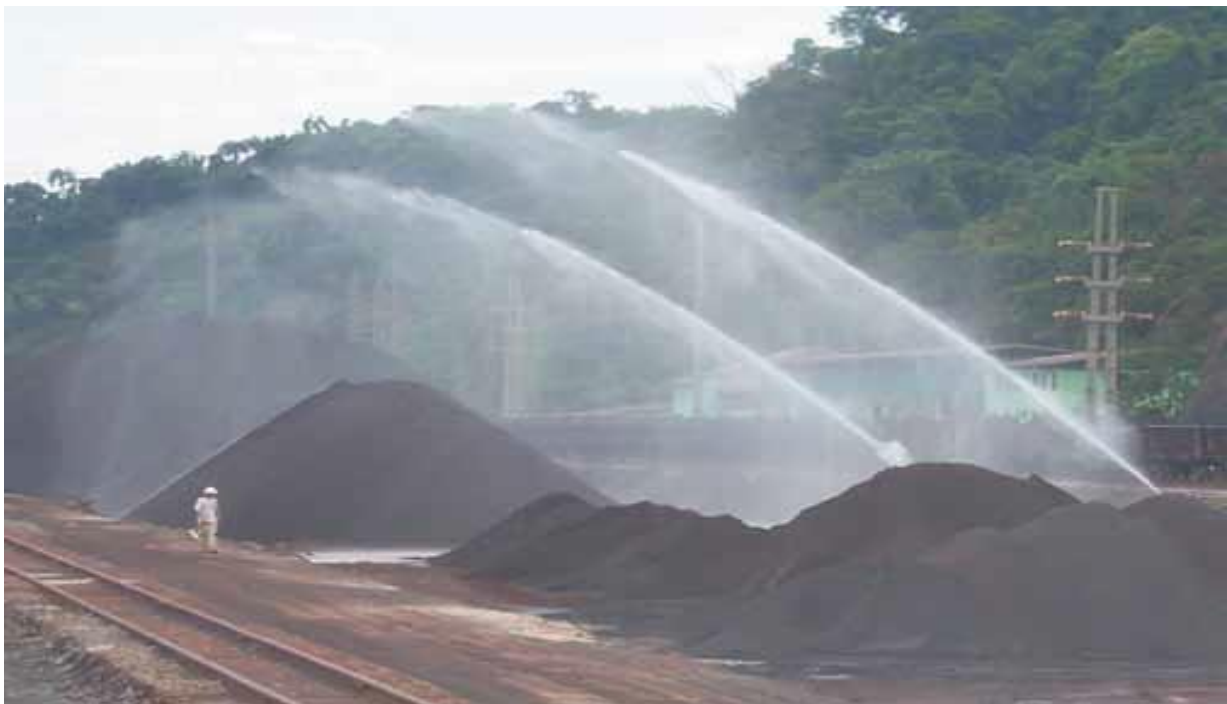
Fig 7.1: Static water sprinkling system in an Australian opencast mine ( http://australianminingreview.com.au/central-control-system-making-dust-control-easy/ )
