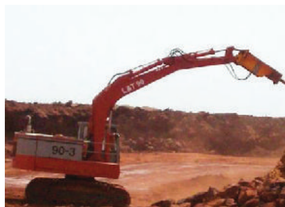
(e) Rock-breaker (120 hp)
