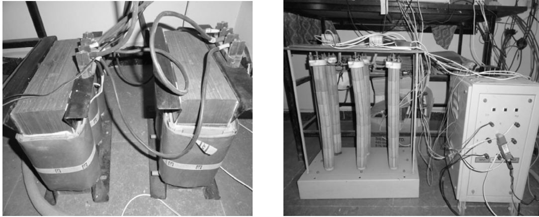
Fig.6.2 Photograph of inductor and resistor load
