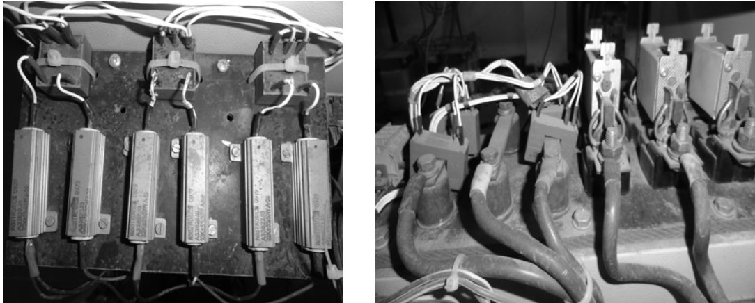
Fig.6.6 Photograph of voltage sensor and current sensor
