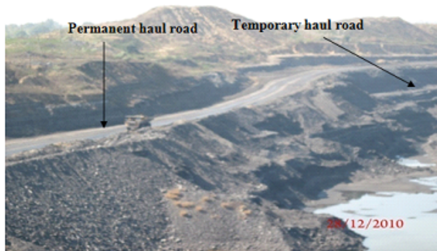
Figure 2.1: A typical mine with permanent and temporary haul roads
