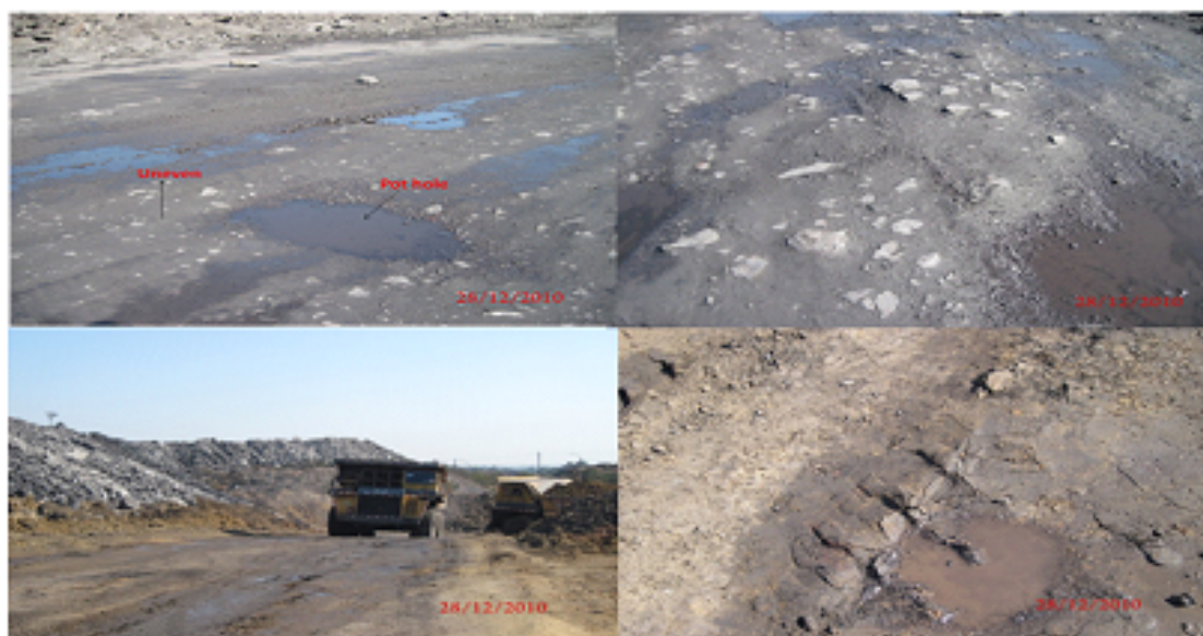
Figure 4.1: Uneven surfaces and potholes observed in the haul roads
