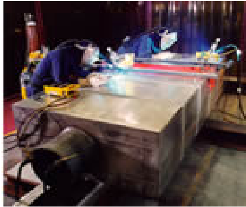
Figure 1.4. Step 4. Welding of nozzles and headers to HX (courtesy HEATRIC™)
