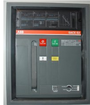
Figure 3.5 Front panel of a 1250 A air circuit breaker manufactured by ABB
