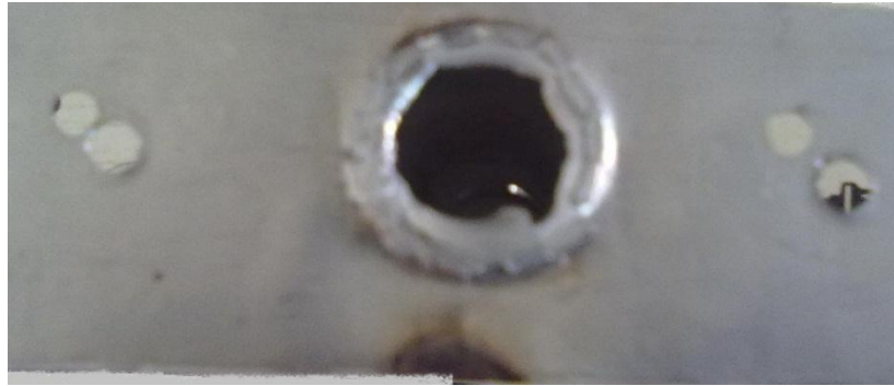
Fig 11 the weld joint between Aluminium pipe and stainless steel plate
