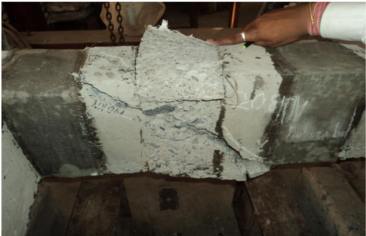
Figure 14 shows the failure pattern of the retrofitted beam, when the GFRP sheet was removed.
