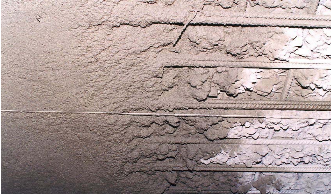
Fig 1.2: concreting of fire damaged slab
