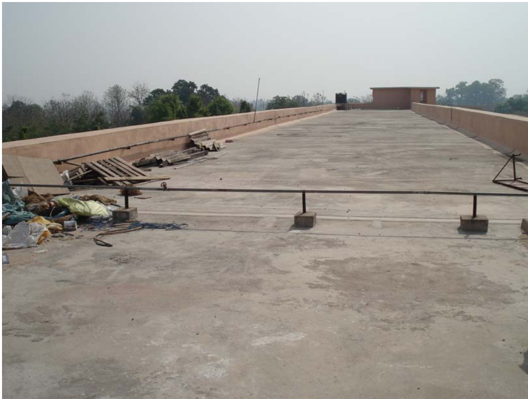
Figure-3.4: Institute main building roof top (photographic view)
