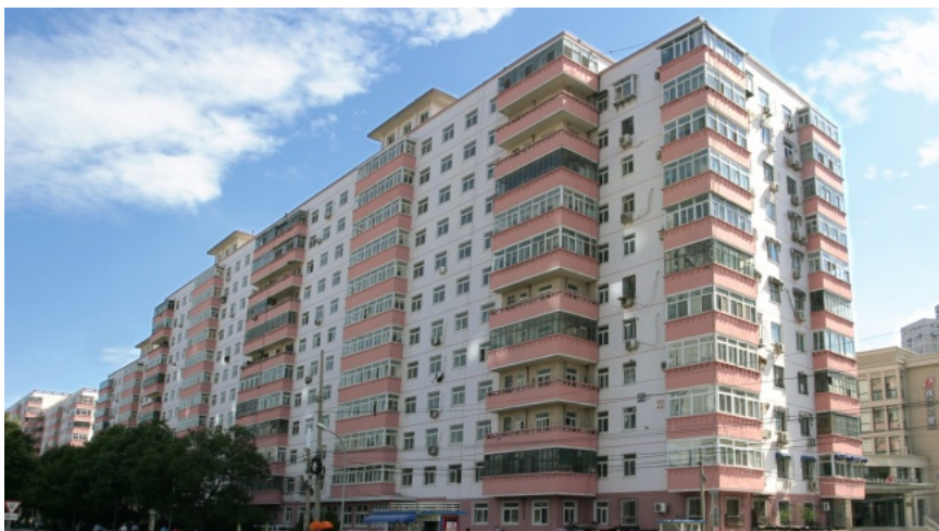
Photo 3-1: precast panel system residential Housing of Qiansanmen in Beijing. source: unknown photographer.
