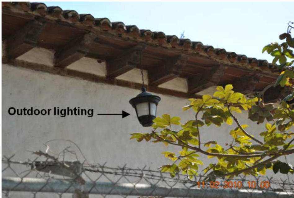
Image 141 418 . Lamp detail of south façade.
