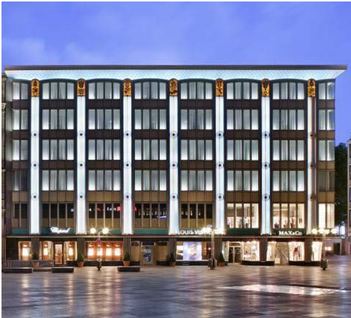
Image 45 174 .Outdoor lighting of Das Blau-Gold-Haus in Cologne, Germany, 2012.
