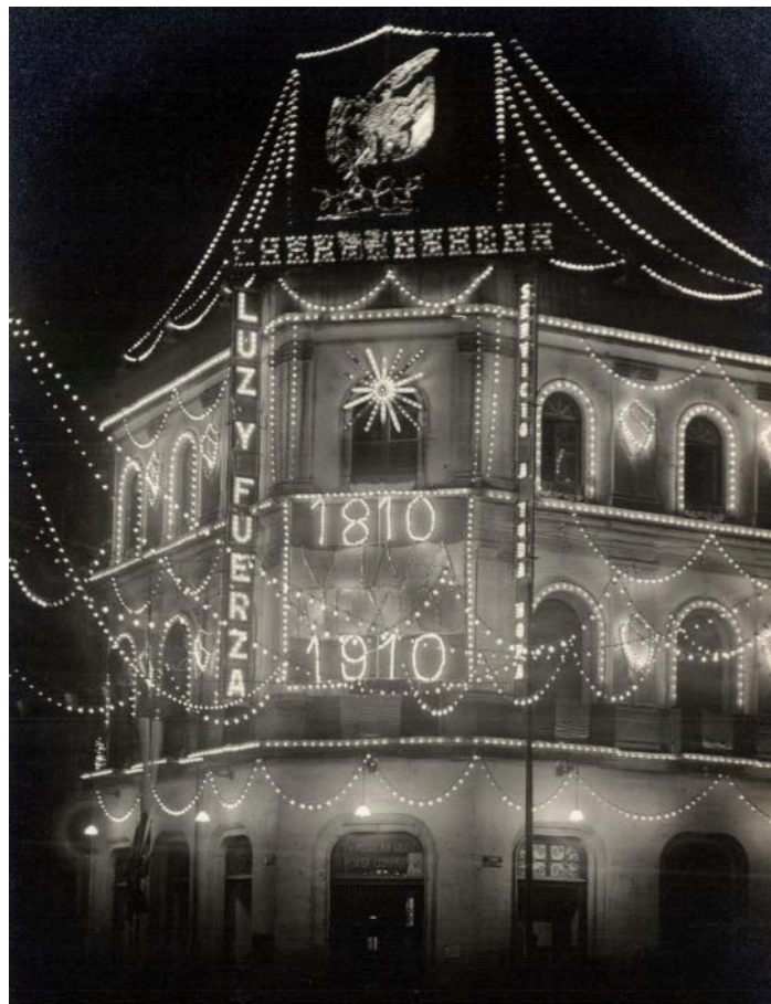
Image 19 106 . The building of Compañía de Luz Eléctrica y Fuerza Motríz , 1910. The moldings which divided the bodies of the building were highlighted. Contour lighting as technique.
