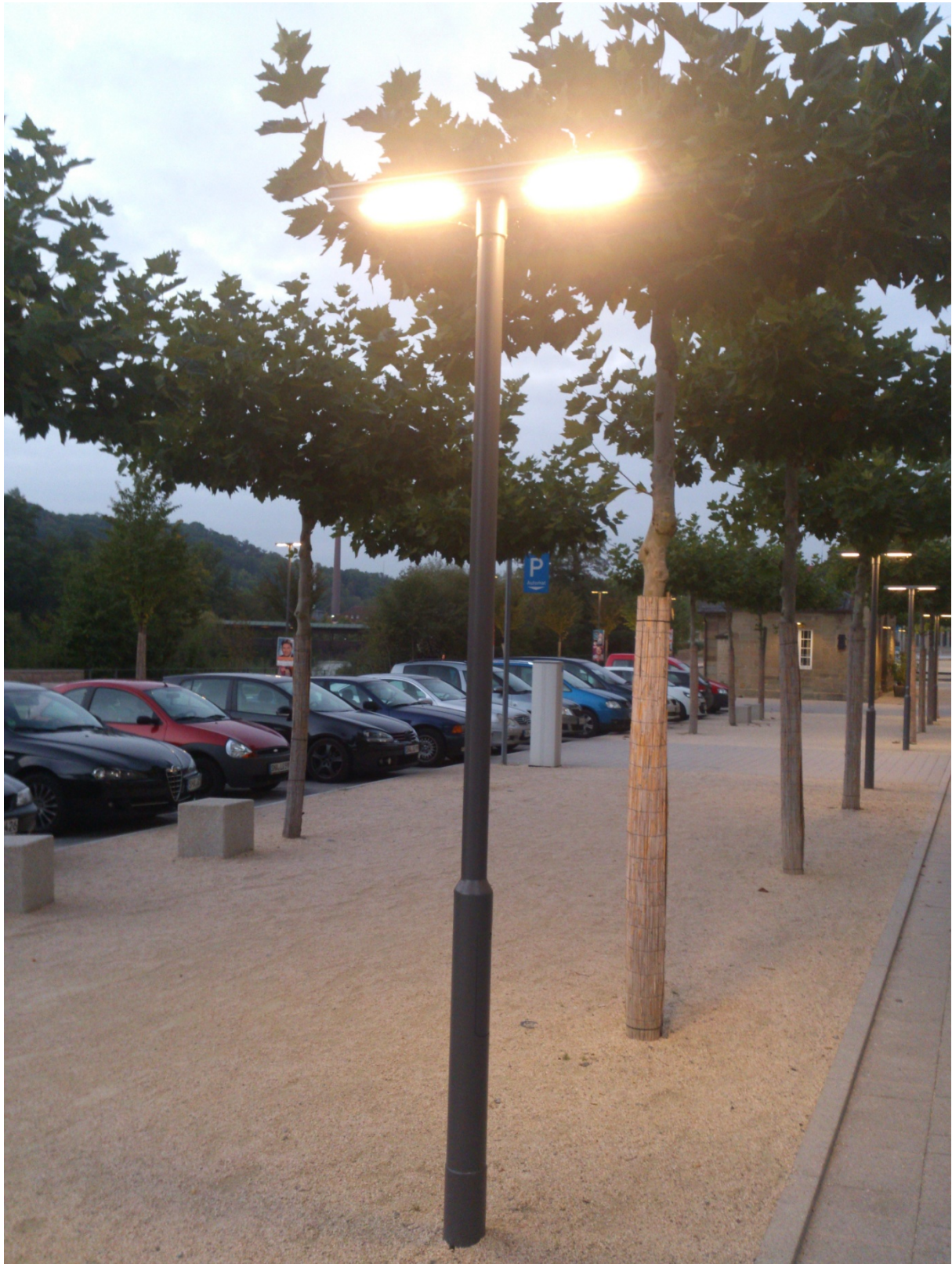
Image 103 306 . Streetlights of Salinenstraße in Schwäbisch Hall, Germany, 2013. The luminaries have amber color, type Siteco SL 10micro 307 .
