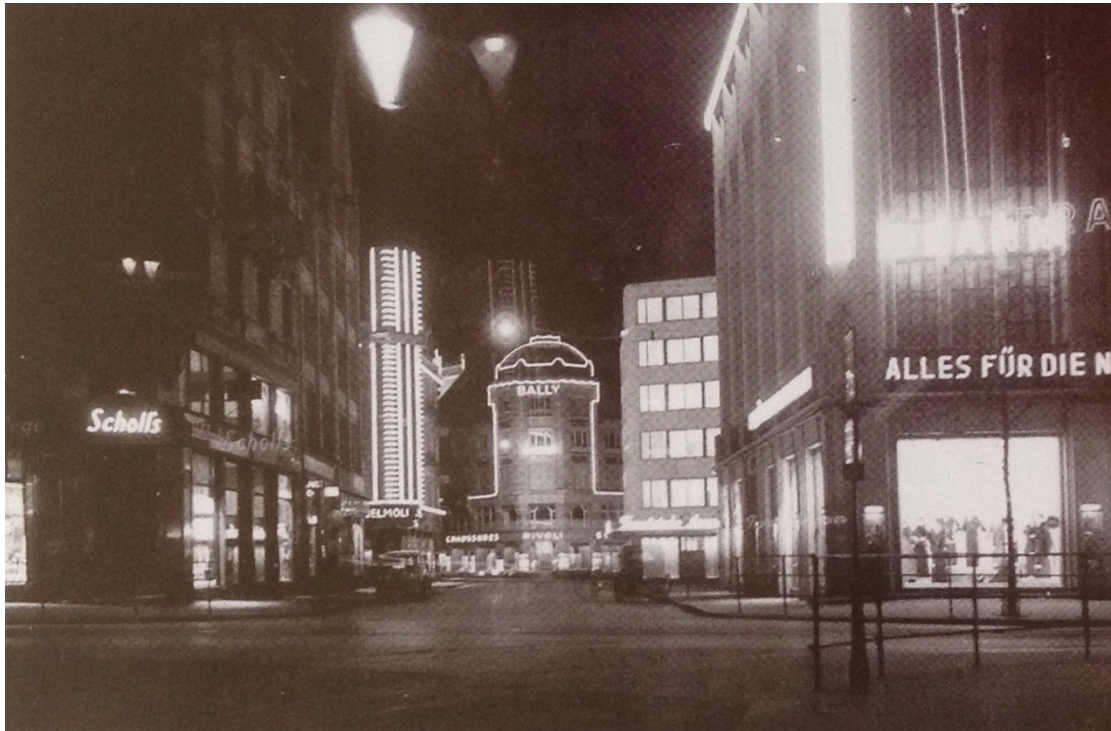
Image 37 147 . Zurich Light-week in 1932. Buildings were illuminated from indoors to outdoors. Contour lighting technique was also used and the store signs with light were placed on the facades.
