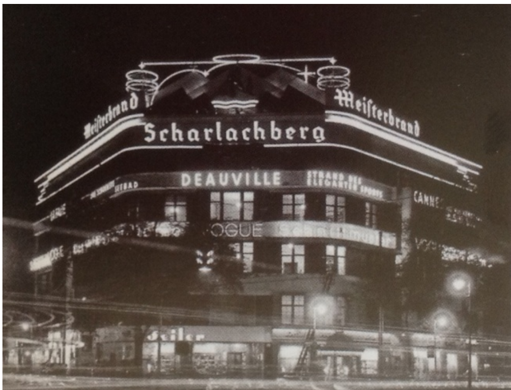
Image 29 126 . Finished work. The photo was taken in 1929.
