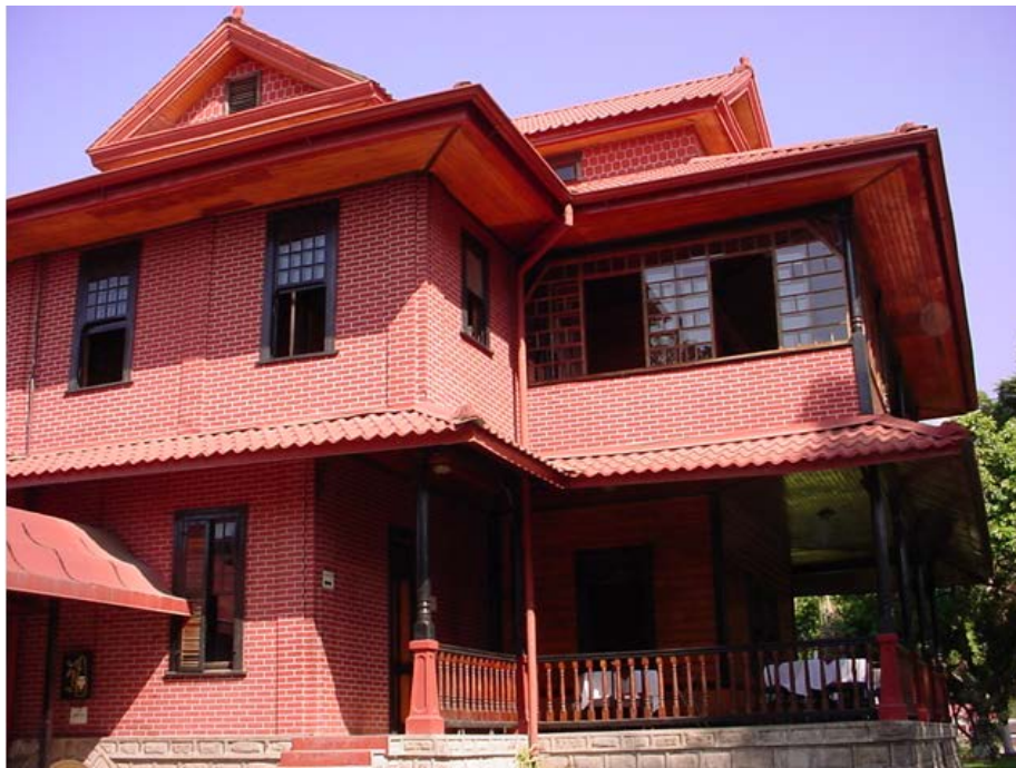
Image 68 240 . Detail of Casa Grande in Santo Domingo, Chiapas, 2010. Artificial textures of walls and roofs that pretend to be bricks and clay tiles. The material used for the walls is a painted zinc-coated steel sheet and for the roofs are prefabricated tiles made of zinc-coated steel.
