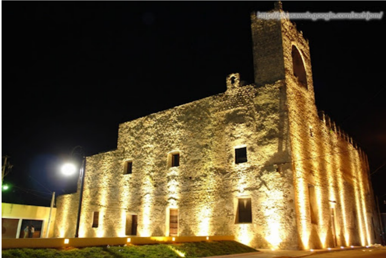
Image 78 255 . Convent of "Tizimin", Mexico. Flat facade with texture. The lighting through projectors placed on the floor of the building, in order to generate an up light, which creates columns of light on the surface of walls.
