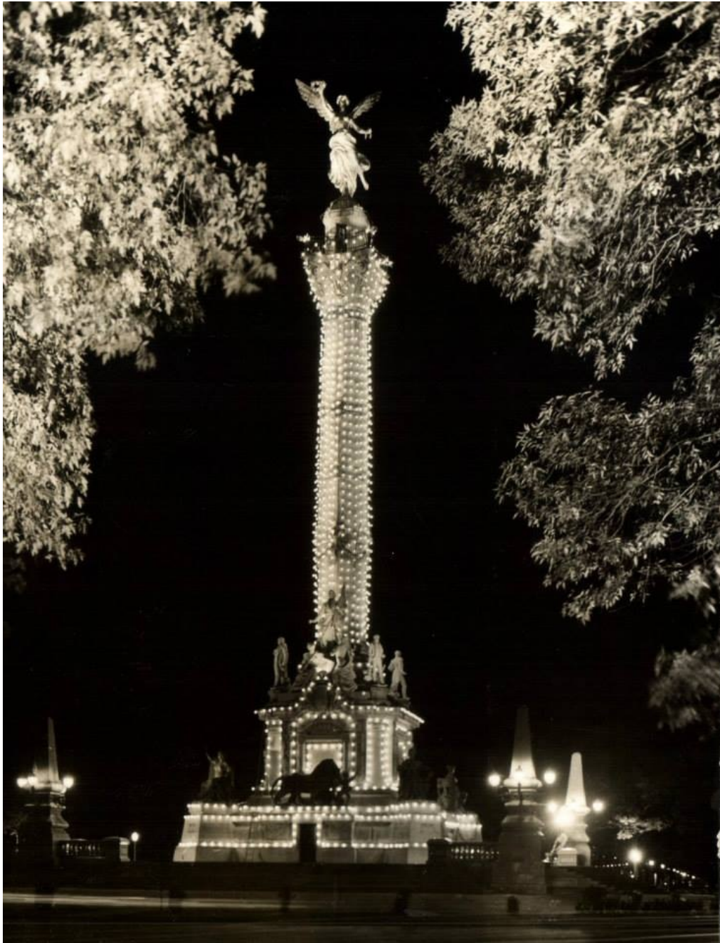
Image 24 116 . Monumento a la Independencia 1910. Technique used was contour lighting and light projection.
