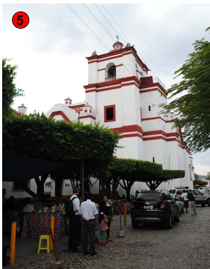
Image 136 412 . Views 5 (see image 131). This photo was taken from “Capitan Vicente López” street to the temple. From this view we can see the monumentality of the bell tower, temple’s north façade, Ficus-trees and some stalls between the street and the temple. This route is the most crowded by pedestrians.
