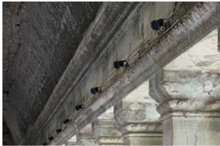
Image 5 34 . Lighting system of Angkor Wat temples. The luminaries are placed at the same distance from each other.
