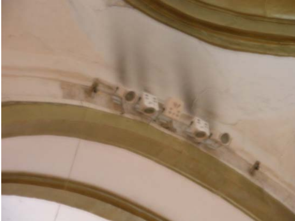
Image 8 38 . Luminaries burned the finish of the spandrel of San Marcos Cathedral (08.12.2008), Tuxtla Gutiérrez, Chiapas.
