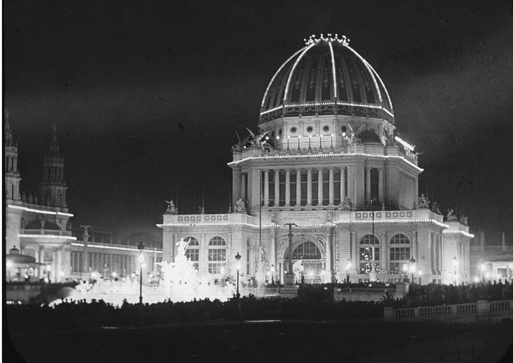
Image 34 141 . The Grand Court of Honor Building at night, Chicago's world fair 1893. Contour lighting technique used to delimiting the heights.
