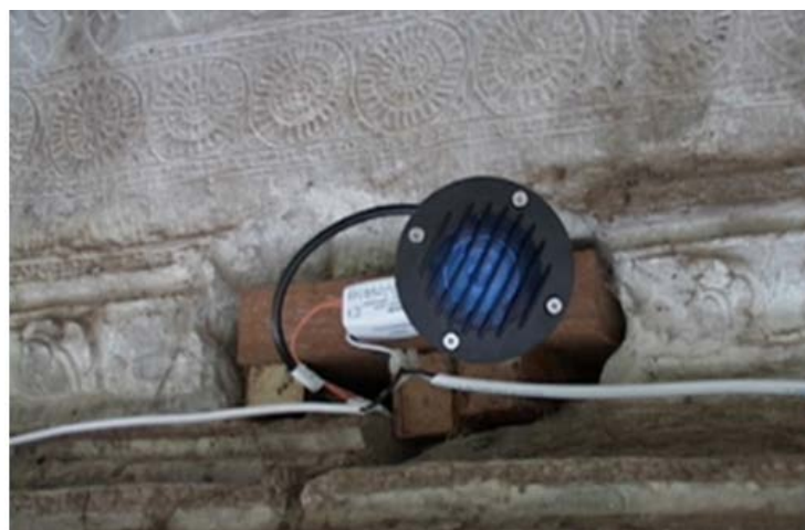
Image 6 35 . Lighting system of Angkor Wat temples. Perforation of a lintel with ornamentation of high reliefs, made in order to place a luminary.
