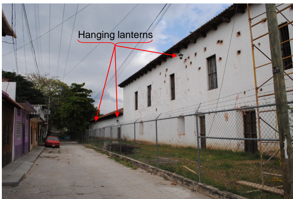
Image 143 420 . Current lighting system on the south façade of the convent. The photo was taken from the street De la Independencia . In this street there are no streetlights, which could illuminate the south façade of the convent.
