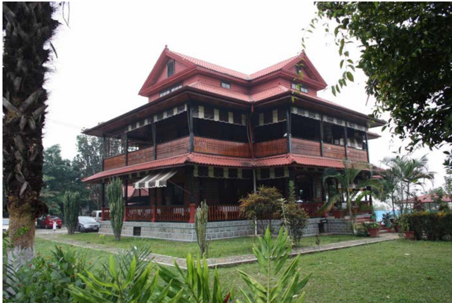
Image 67 239 . Complet view of Casa Grande in Santo Domingo, Chiapas, 2010. Built in 1920s.
