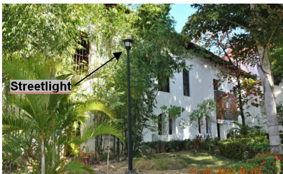
Image 144 421 . East façade of the convent. There is only one source of light that illuminate the eastern façade, which we can see in this photo. The streetlight has a fluorescent lamp of 100 watts with classic diffuser. However it is insufficient to light this façade and the front yard.
