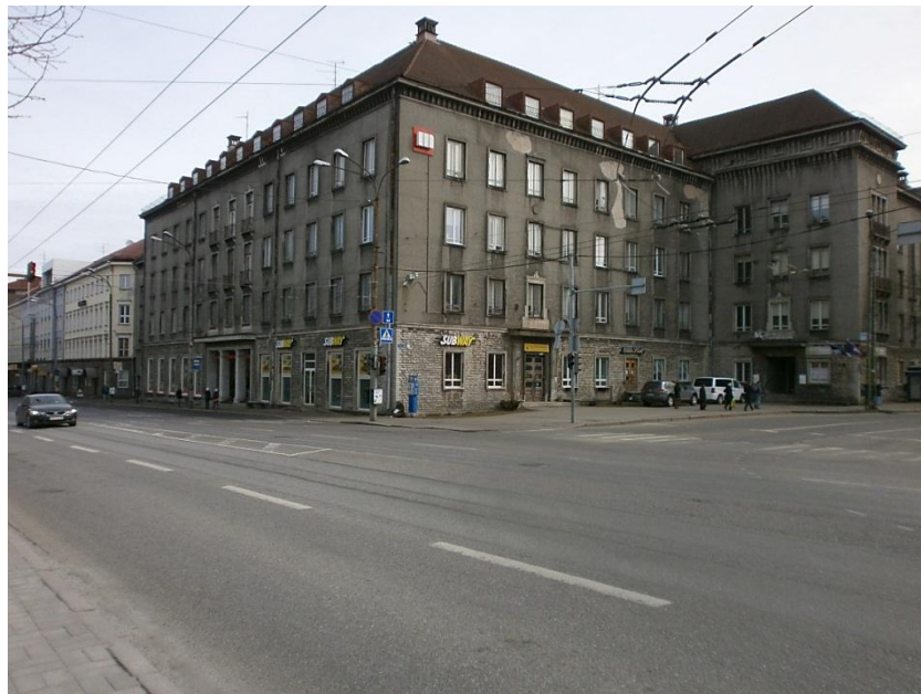
The Estonia Boulevard administrative buildings in Tallinn that date to the turn of 1940s and 1950s. The urban spatial design was created by Harald Arman and the foregrounded building by Enn Kaar. (The author).
