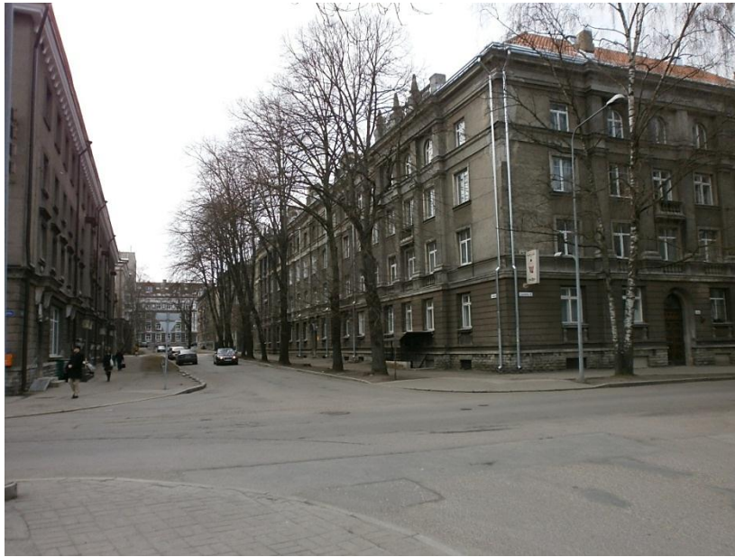
Apartment buildings at the corner of the Kauka and Lembitu streets in Tallinn that date to the turn of the 1940s and 1950s. (The author).
