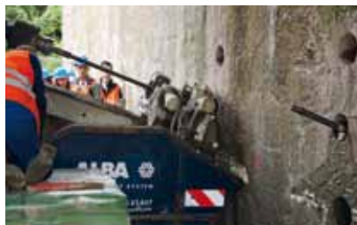
d) Strengthening of the abutment by anchors
