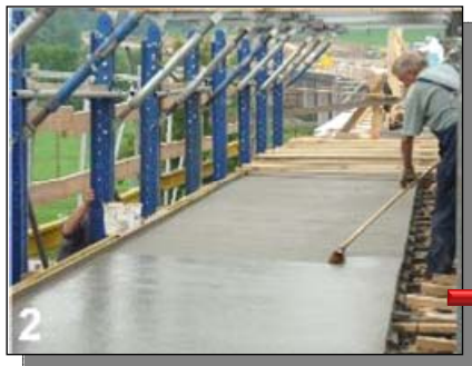
documentation of construction site
