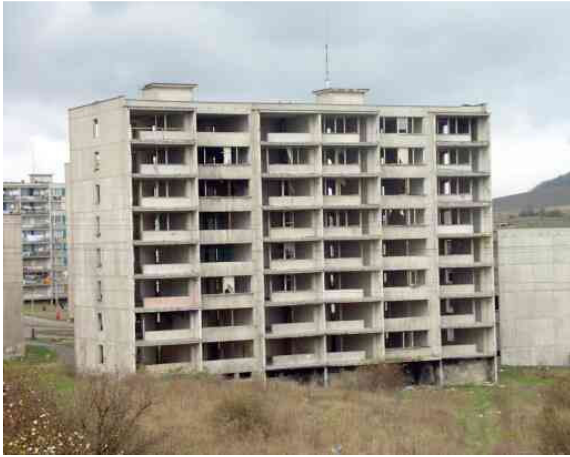
Figure 3: The building to be deconstructed
