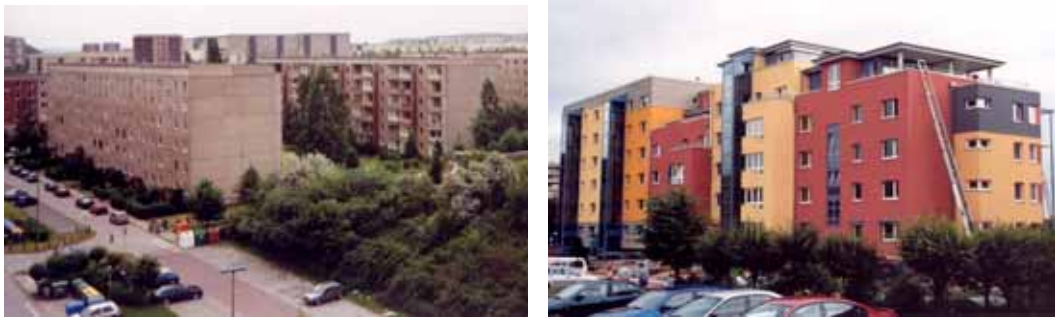
Figure 1 Panel structures before and after revitalization
