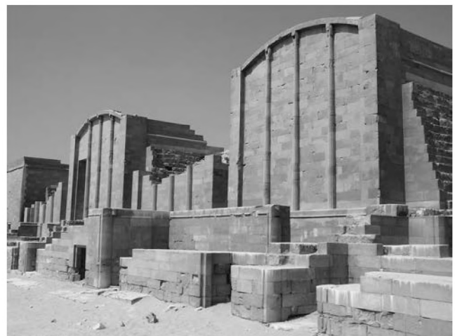
Fig. 4. Cult chapels reconstructed inside Step Pyramid temenos. All these structures were cased by small blocks of the white compact limestone, whereas interior was built with local sandy and marly limestone (photo F. Welc).
