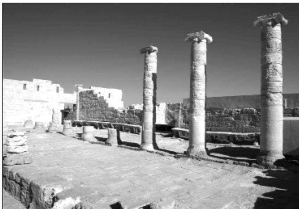
Fig. 10. Columns of the south portico restored, view from the northwest (Photo P. Zambrzycki)
