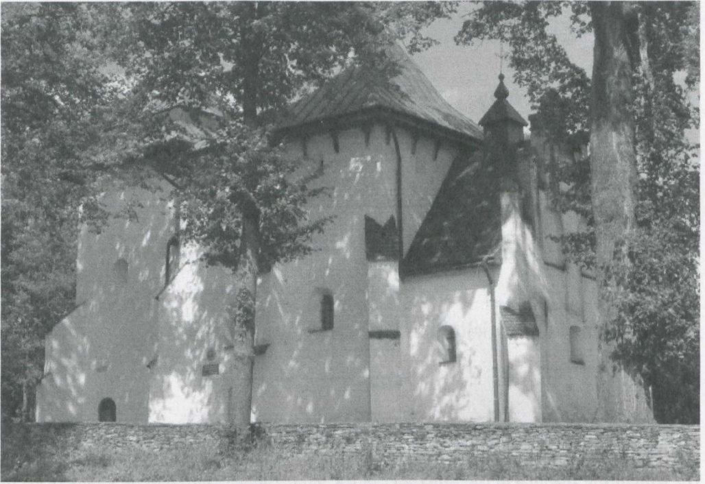
Fig. 1. Posada Rybotycka, St. Onuophrios' church in, the main view (all photos by Piotr Krawiec)
