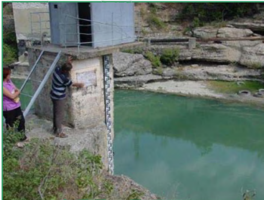
Figure 5: The sign shows maximum historic level of Vjosa River
