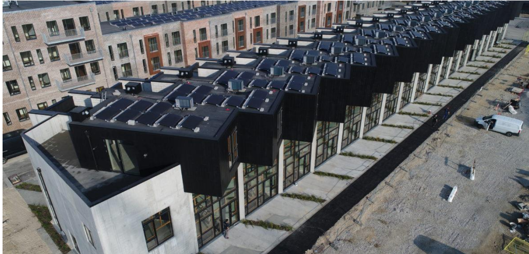
Figure 14: Receiver building (Upcycle Studios) in Case C. (NREP, 2021)
