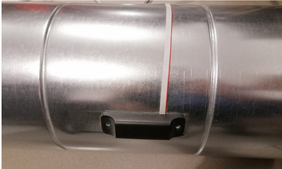
Figure 3.14. Ultrasound device integrated to Ultra Ulsa
