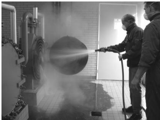
Fig. 1. Cleaning of heat exchanger using low pressure.
