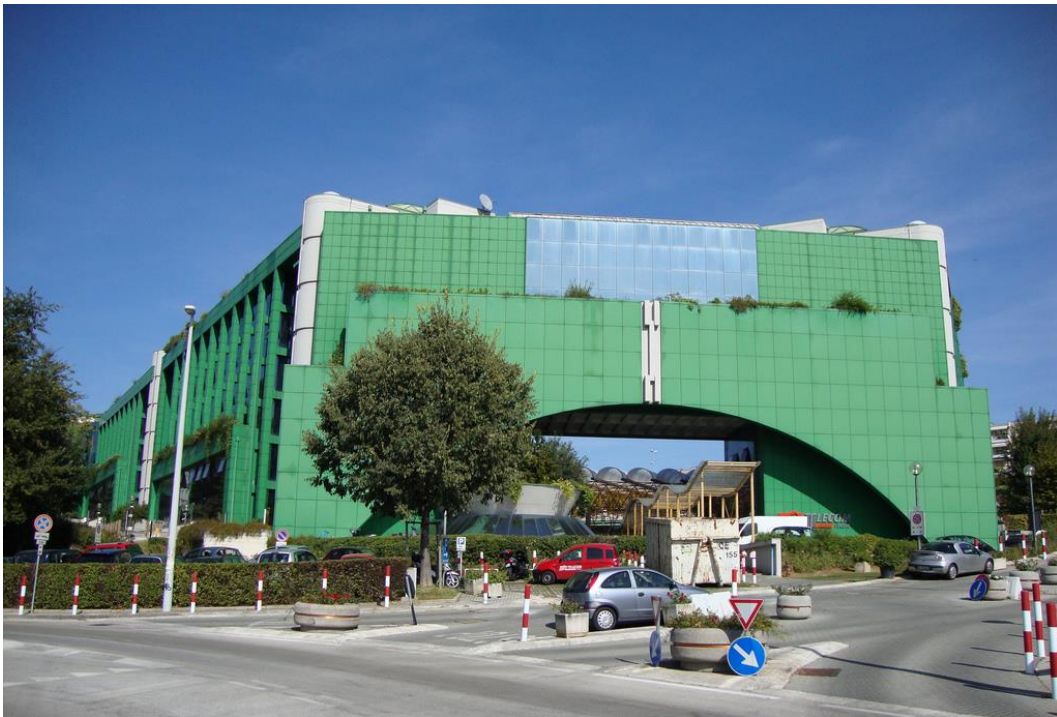
Figura 4. Administration Center of the National Telephone Company, Italia.
