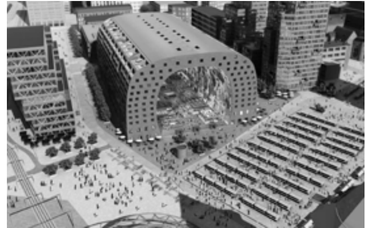
Figura 52: Vista exterior de MARKET HALL BY MVRDV
