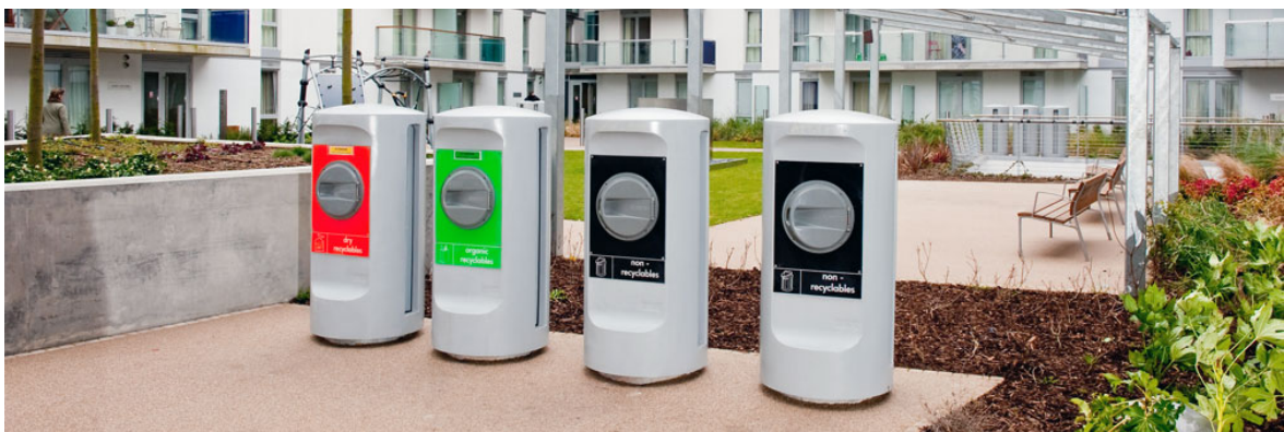
Figure 6-13: Pneumatic collection inlets (BWC WM 5.5.1) are emptied automatically when full or at times. 1 each 150-250 people at streetscape, indoors floor, doorway, street level or outdoors, wall-mounted as well as freestanding. Pneumatic system needs for infrastructural intervention in district underground and, for this reason, only bio-waste collection would not be cost effective if not connected to other waste streams
