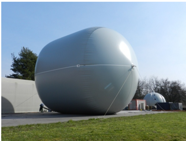
Figure 6-24: gas bag (BP GS 2.3) is external to digester to compensate biogas fluctuations
