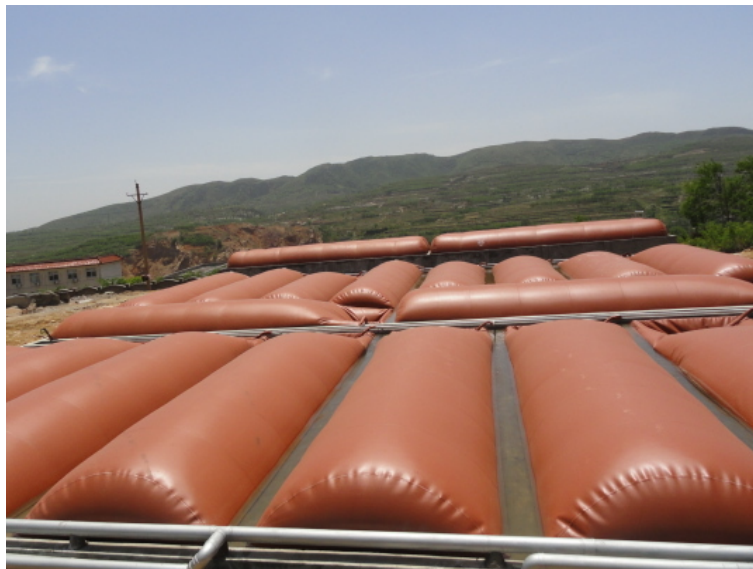
Figure 6-20: rubber-balloon reactor (BP DR 1.1) is an off-ground digester simple and cheap, that achieves high temperature under sunny sky and is easy to clean and empty. Being an inflatable balloon exposed to natural event, possible damaged has a short life span
