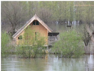
House flooded near the forest of Caraorman
