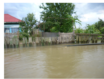
Flooding the main street of the locality of Carorman (b)
